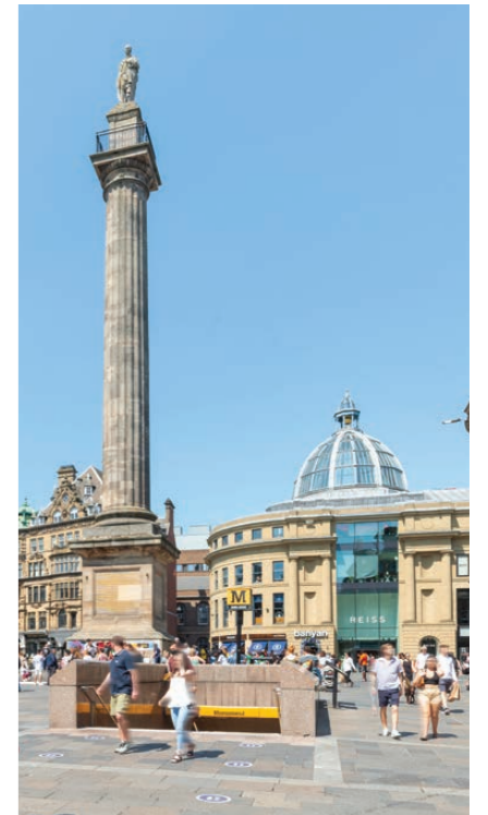
Monument Metro Station
