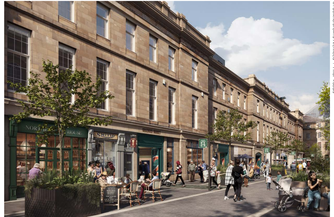
CGI of Grainger Market Regeneration on Nelson Street, due to complete Spring 2025.
